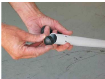
Installing end plugs
