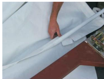
Insert tensioning tubes
